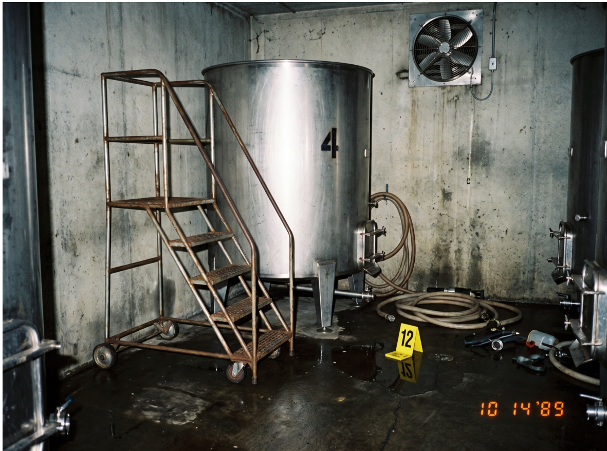
89-1013-A · Roll 1 Fr. 4 · Tank room, Tank 4 and platform, looking N. Fan on E wall running. 0705 hrs. - Ortiz
